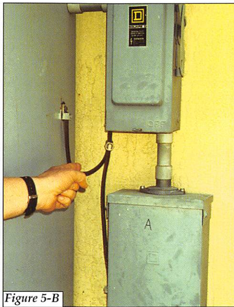
Figure 5. The service entrance (Figure 5-A) and sub-panels (Figure 5-B) are bonded to a buried 4/0 copper ring-ground, as are all other exterior metal objects, including downspouts (Figure 5-C). Note the large TVSS beneath the middle panel in Figure 5-A.
