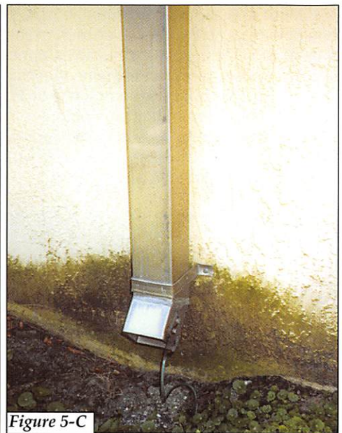
Figure 5. The service entrance (Figure 5-A) and sub-panels (Figure 5-B) are bonded to a buried 4/0 copper ring-ground, as are all other exterior metal objects, including downspouts (Figure 5-C). Note the large TVSS beneath the middle panel in Figure 5-A.
