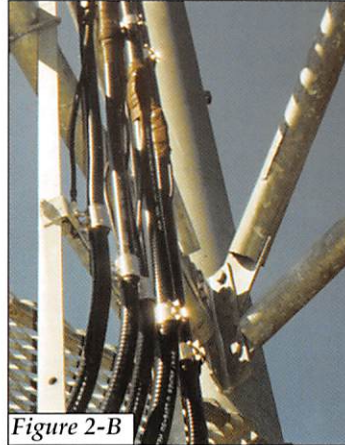
Figure 2. Braided, tinned-copper #29X lightning cables are soldered to the shields of coax cables ( Figure 2-A ). The #29X leads are bonded to 4/0 copper cables, which are connected to a horizontal bus on the tower structure ( Figure 2-B ). John West, Power & Systems Innovations, Inc. (PSI), indicates where a length of bare 4/0 copper extends downward to a grounding electrode located directly below ( Figure 2-C ).
